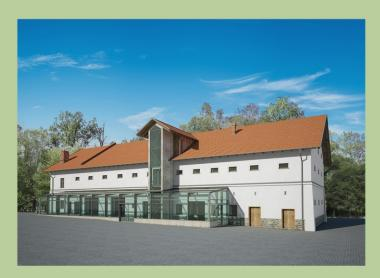
The granary is a plastered brick and stone building with an elongated rectangle layout, divided by a simple bracketed cornice above the ground floor, and with a separate pedestal at the bottom, which is raised following the slope of the area. In the internal layout of all the floors, the building features a separated northern part of the proper granary and a smaller southern part, after a major reconstruction in the post-war period.
